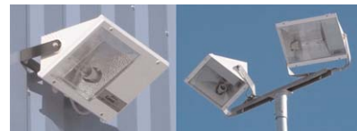
Thorlux AZMET 70 (left) and AZMET 3 (right) used to illuminate the exterior of the building
